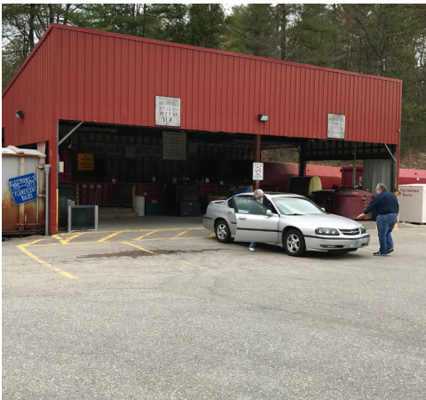
BUILDING EXTERIOR/SIDE & REAR
