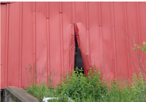
OPENING IN METAL PANEL SIDING
