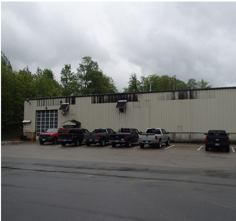
BUILDING EXTERIOR/SIDE & REAR
