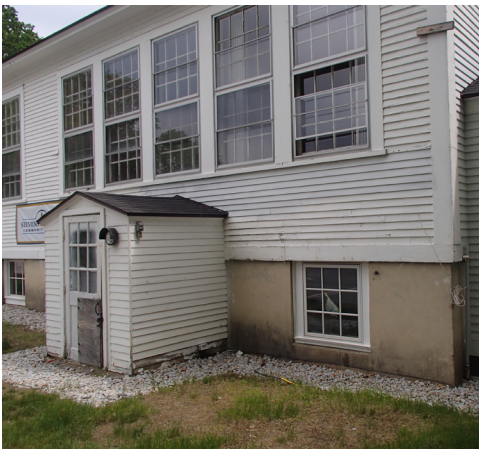
BUILDING EXTERIOR/SIDE & REAR
