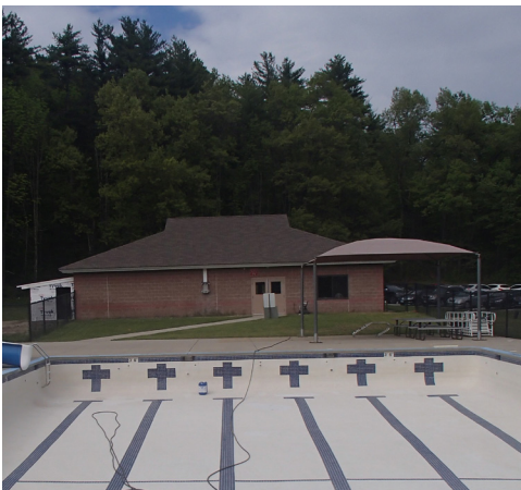
BUILDING EXTERIOR/SIDE & REAR
