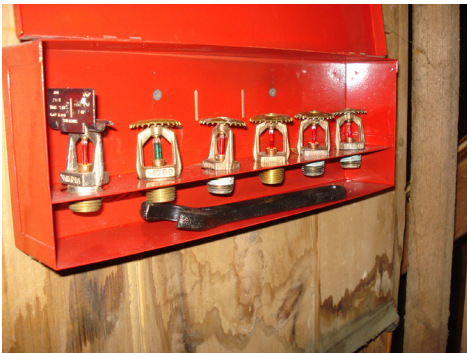
HISTORIC SPRINKLER HEADS
