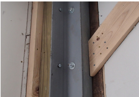
STRUCTURAL REINFOR CONCRETES AT SOUTH WALL
