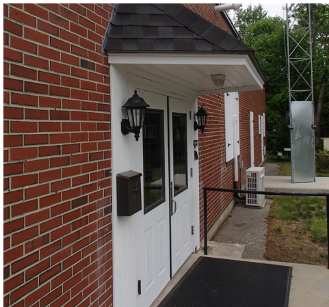
BUILDING EXTERIOR / SIDE & REAR
