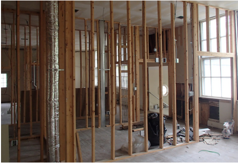
TYPICAL INTERIOR CONSTRUCTION
