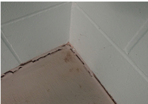
SEPARATION AT WALL AND FLOOR
