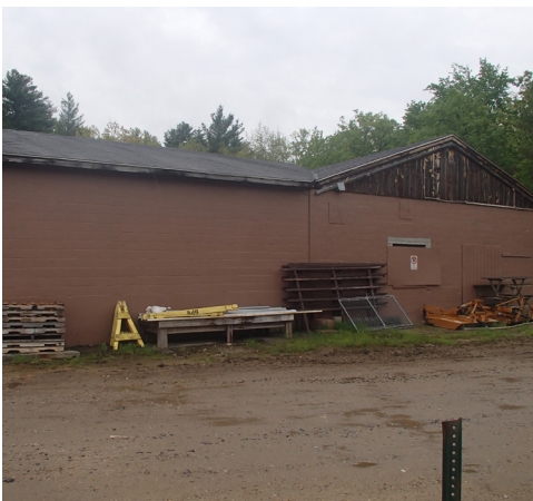
BUILDING EXTERIOR/SIDE & REAR
