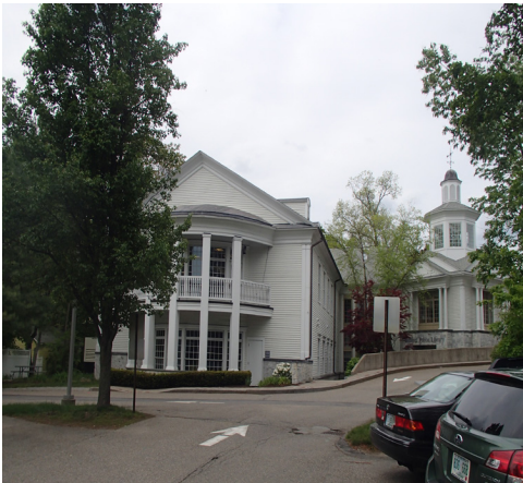
BUILDING EXTERIOR / SIDE & REAR
