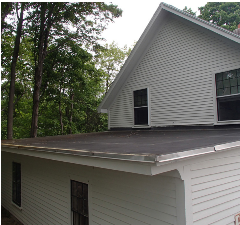
BUILDING EXTERIOR / SIDE & REAR
