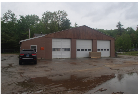
DIRT AND PUDDLING AT SITE
