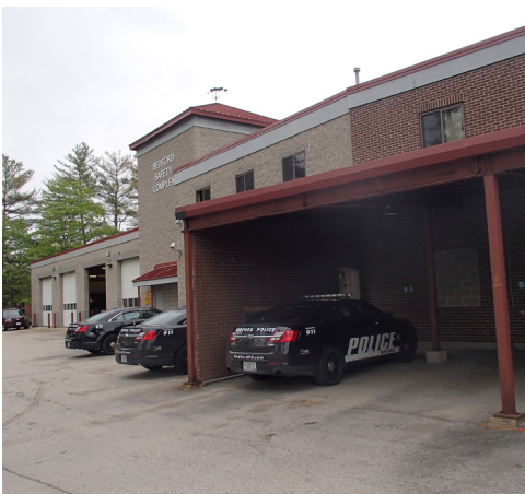
BUILDING EXTERIOR / SIDE & REAR
