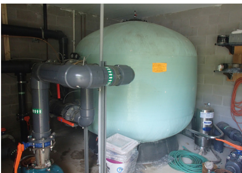
POOL FILTERING EQUIPMENT
