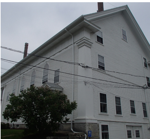
BUILDING EXTERIOR/SIDE & REAR
