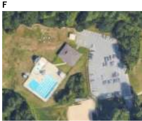
F Pool Facility 20 Country Rd.
