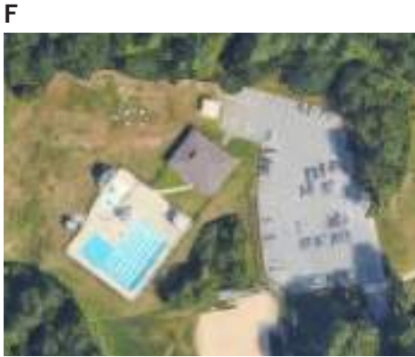
F Pool Facility 20 Country Rd.
