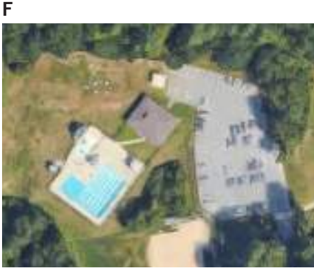
F Pool Facility 20 Country Rd.
