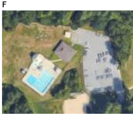
F Pool Facility 20 Country Rd.
