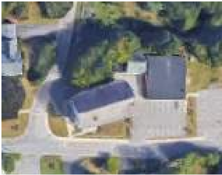
BCTV & BCTV Annex 10 Meetinghouse Rd
